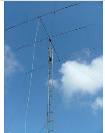
The classic tri-band HF beam with a rotator (also known as Armstrong rotation).
